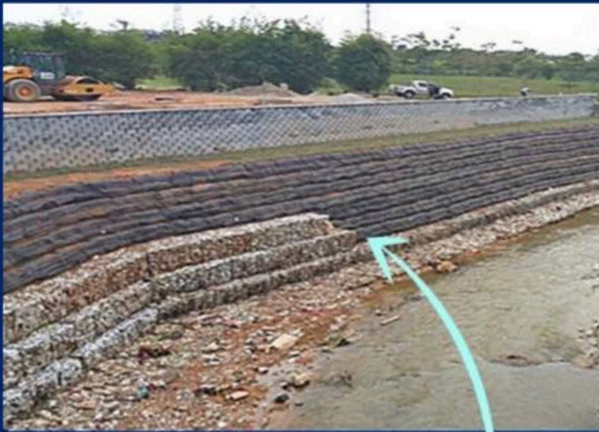
Gabion and Mattress Project in Selangor
