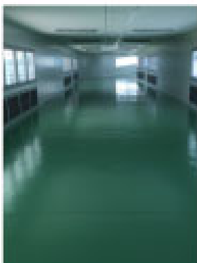
Epoxy floor coating
