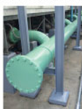
Polyurethane pipes coating (uv-protection)
