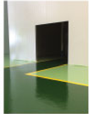
Epoxy floor coating with safety line
