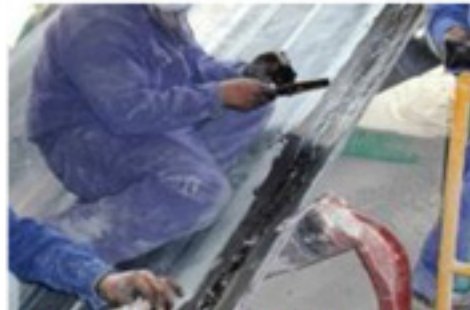
Repair surface of the rubber belt
