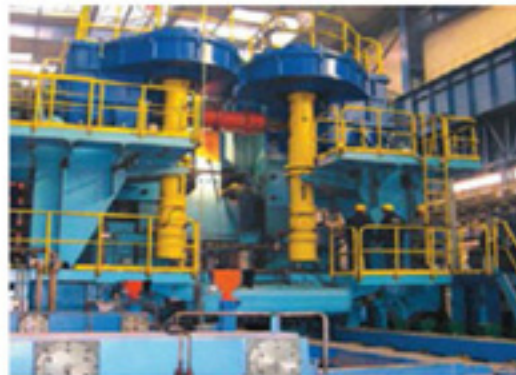
Rolling mills (vertical rolling stand)
